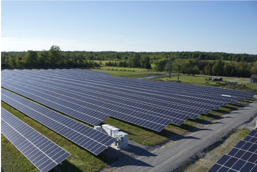
Image 4.2: Typical Fixed Panels (with Conversion Unit/Inverter)
